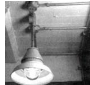
Typical Class 1 Div 1 conduit installation
